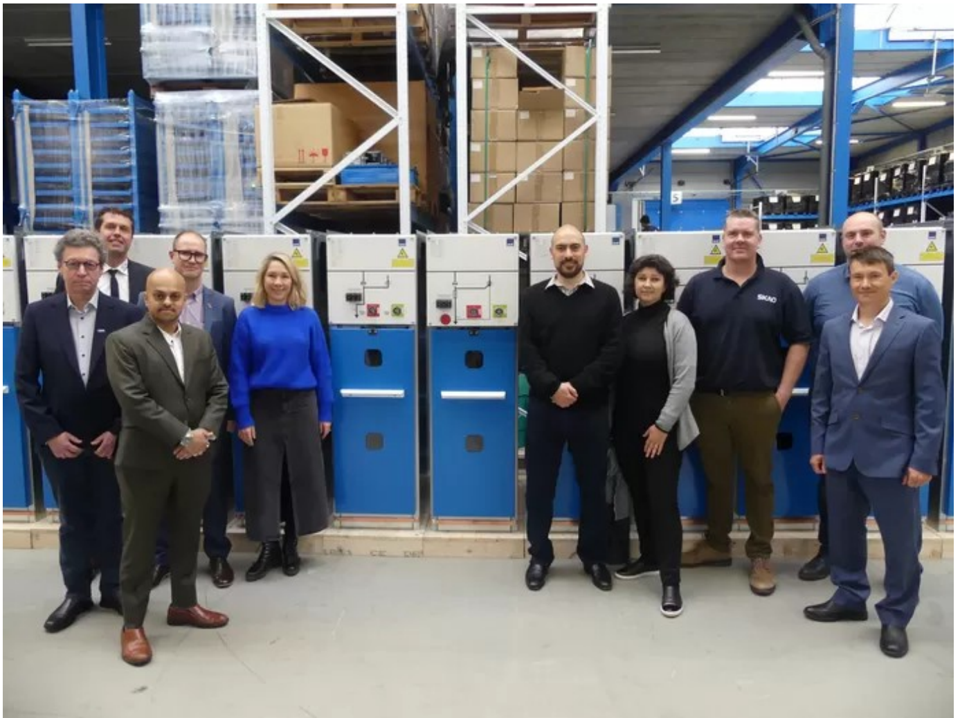
SwitchGear Company's cells were inspected Monday by SKAO and NHP representatives. © Anthony Stadius
