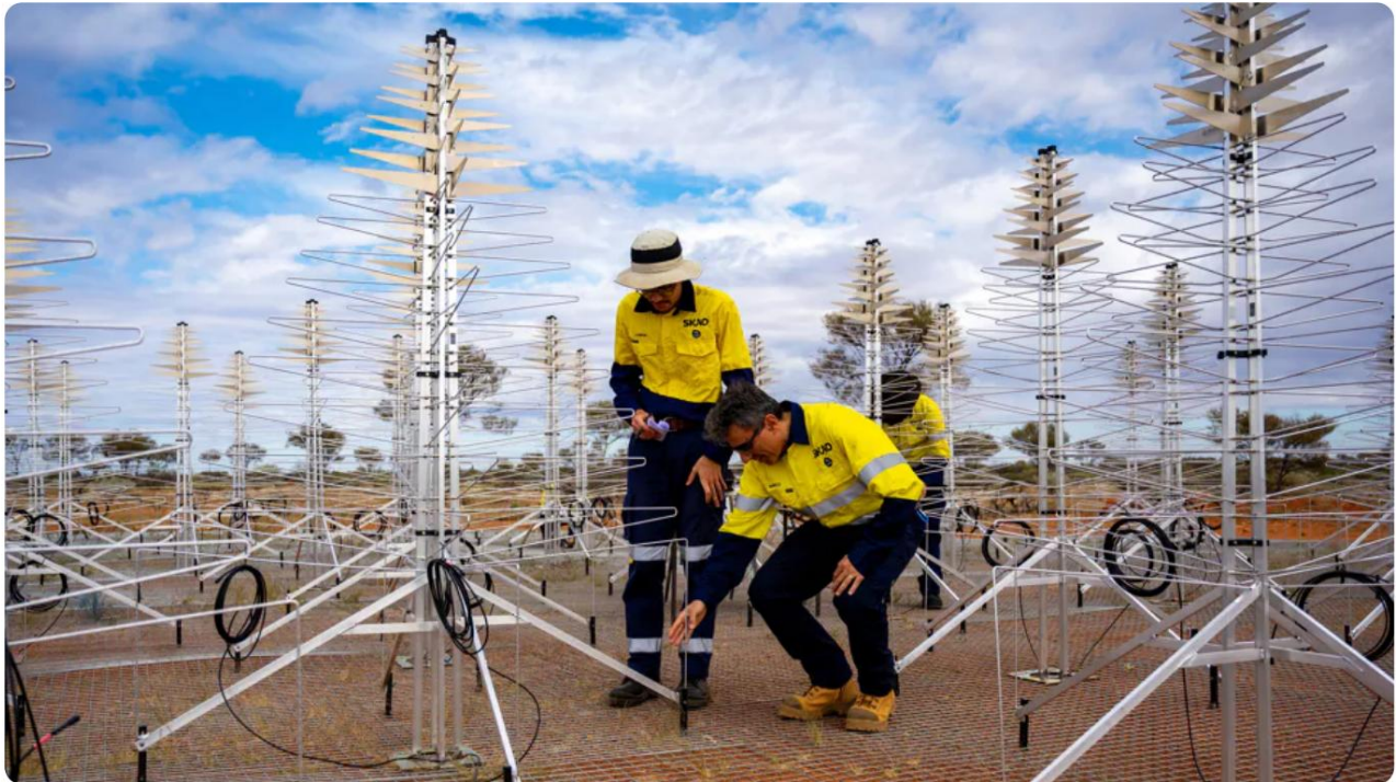
The first antennas are already being installed in Australia ©SKAO
